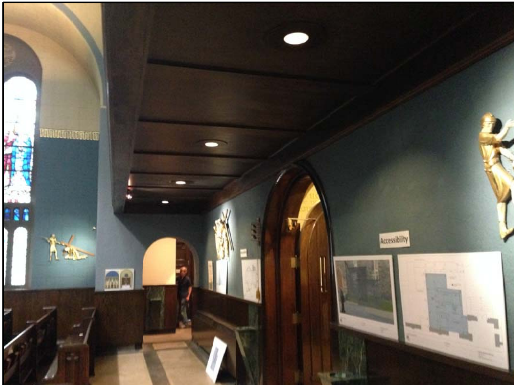
IMAGE 2/A3.17 EXISTING NAVE
